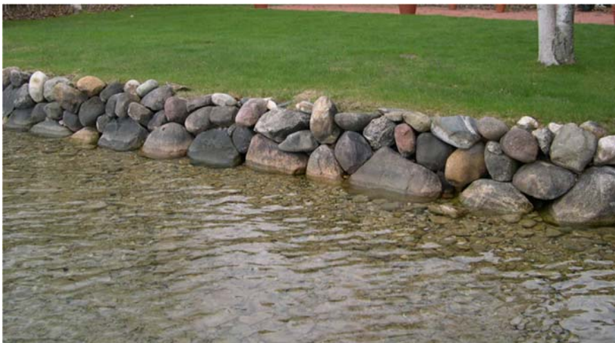
Revetment. Photo Credit: Tip of the Mitt Watershed Council
